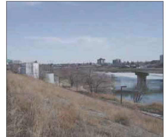
Undeveloped riverfront land and sewage pump station.
