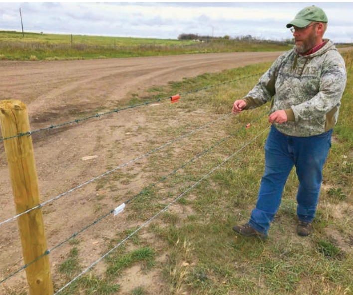
Resource Management Officer Renny Grilz installing wildlife friendly fencing tabs in the Northeast Swale
