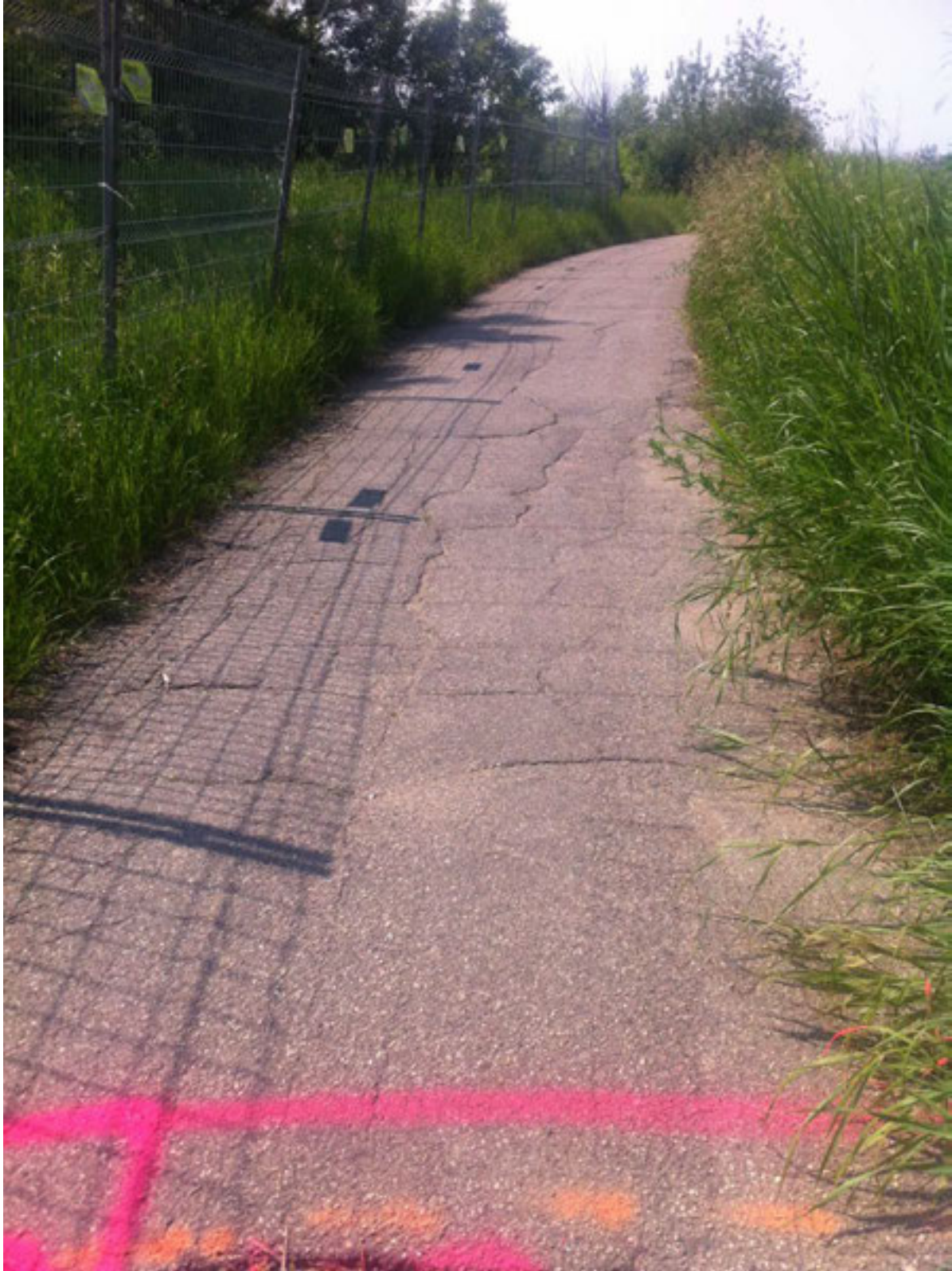
Image 6 – Block Cracking (University of Saskatchewan)
