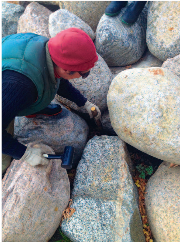
Above: Meewasin's Horticulturalist Foreman Kathy Thomas, "Willow Staking" as part of the armoring of the Shakespeare Site on the South Saskatchewan River
