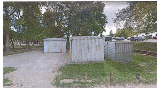
Existing sheds at Kinsmen Park.
