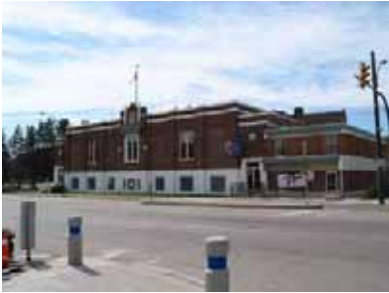
Figure 4: The Royal Canadian Legion Building within CCZ at end of 2 nd Avenue.
