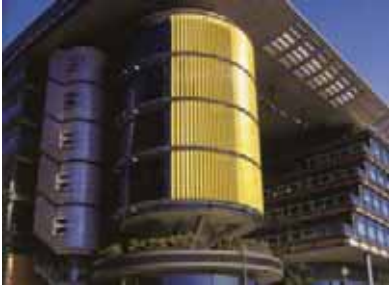
Figure 31: An assemblage of independent volumes into one building assists in breaking down the apparent mass.
