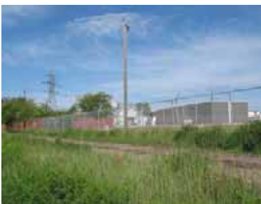
Figure 15: Existing electrical substation to remain at end of Avenue C.
