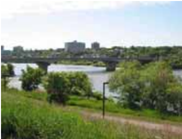
Figure 16: Riverbank Park – west side of Senator Buckwold Bridge looking southeast.
