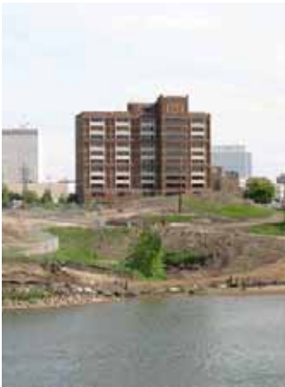
Figure 22: RPCZ at east side of Senator Buckwold Bridge looking north. Clinkskill Manor in background (CCZ).
