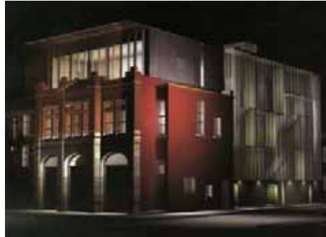
Figure 66: Variety in material and colour is achieved through renovation.
