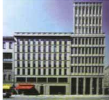
Figure 32: Regular rectilinear volumes masonry cladding and small punched openings give the buildings an appearance of greater mass.
