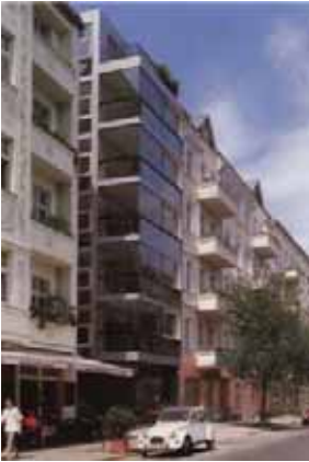
Figure 65: Variety in fenestration and style is achieved through infill construction.
