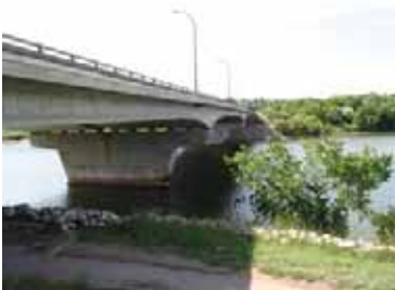
Figure 18: West side of Senator Buckwold Bridge looking south.
