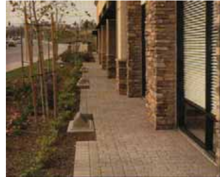
Figure 74: An example of building lighting integrated into a public walkway.
