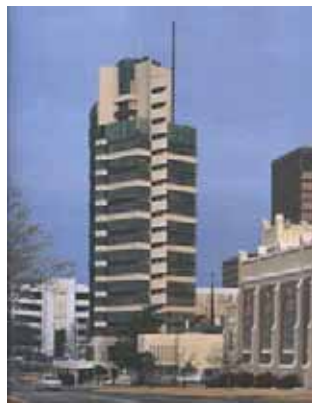
Figure 29: Sample of hotel tower.
