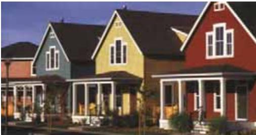
Figure 56: Historically proportioned row housing would blend with Riversdale but would have to meet the theme.
