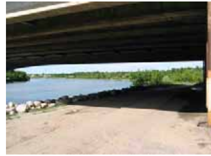
Figure 23: Existing pedestrian underpass below Senator Buckwold Bridge looking west.
