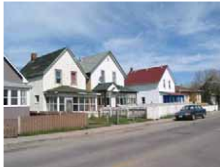
Figure 8: Streetscape across Avenue C from RCZ.
