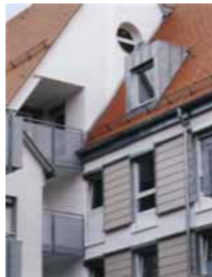
Figure 39: Sloped metal roofing system.
