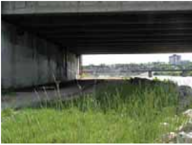
Figure 20: West side of Senator Buckwold Bridge looking east under bridge.
